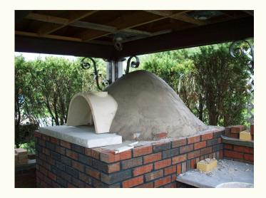
8) A door-without-a-hinge or entrance cover for the oven entrance is provided. It can be propped up slightly (to provide combustion air) at the outside of the entrance when a fire is burning in the oven and can be pushed in farther to close off the flue to keep the oven warm longer after the fire has burned out.
