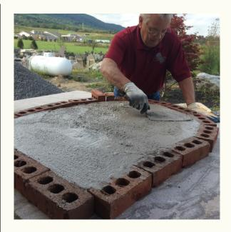
3) Lay out a 24" circle on oven floor and set the entrance tunnel and 14 firebrick as shown using HeatStop II refractory mortar.
