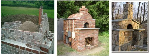
7) The 4"x8" flue liner should be enclosed within a chimney with walls at least 4" thick of solid masonry. If the chimney is inside a house it must conform to all applicable codes dealing with clearance to combustibles and height above the roof. If the oven is outside the flue need only be enclosed in masonry as high as is desired and clear of combustibles.
