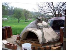
6) If the oven is associated with a cooking fireplace or is part of a larger chimney mass, brick can be laid directly on the insulating concrete. If the oven is to stand alone it can be stuccoed, plastered or finished with any non-combustible masonry material such as tile. brick or stone.
