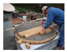
3) Lay out a 36" circle on oven floor and set the entrance tunnel and five base sections using HeatStop II refractory mortar.
