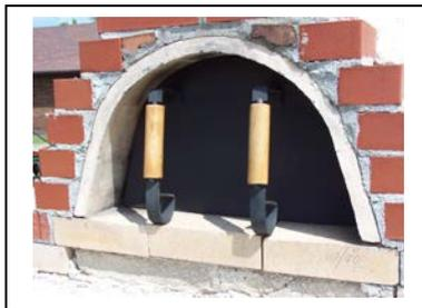
8) An entrance cover for the oven entrance is provided to help keep the oven warm. It can be propped up slightly (to provide combustion air) at the outside of the entrance when a fire is burning in the oven and can be pushed in farther to close off the flue to keep the oven warm longer after the fire has burned out.
