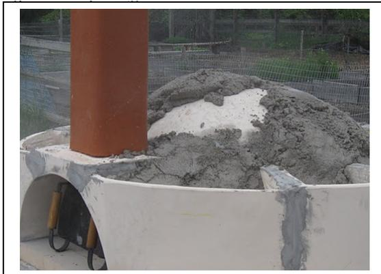
3) Set wall sections (8 pcs) and the entrance tunnel (3 pcs) as shown using HeatStop II refractory mortar.
