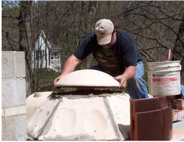
4) Set the oven dome on top of the base sections in HeatStop II refractory mortar.
